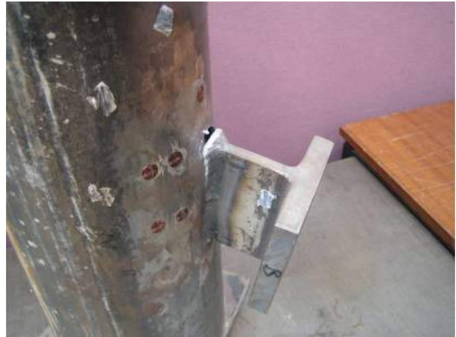
Failure mode (b)
