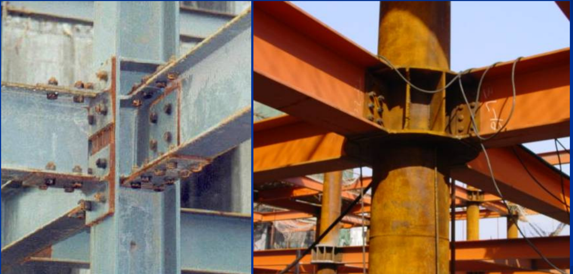
Typical beam-column connections in China
