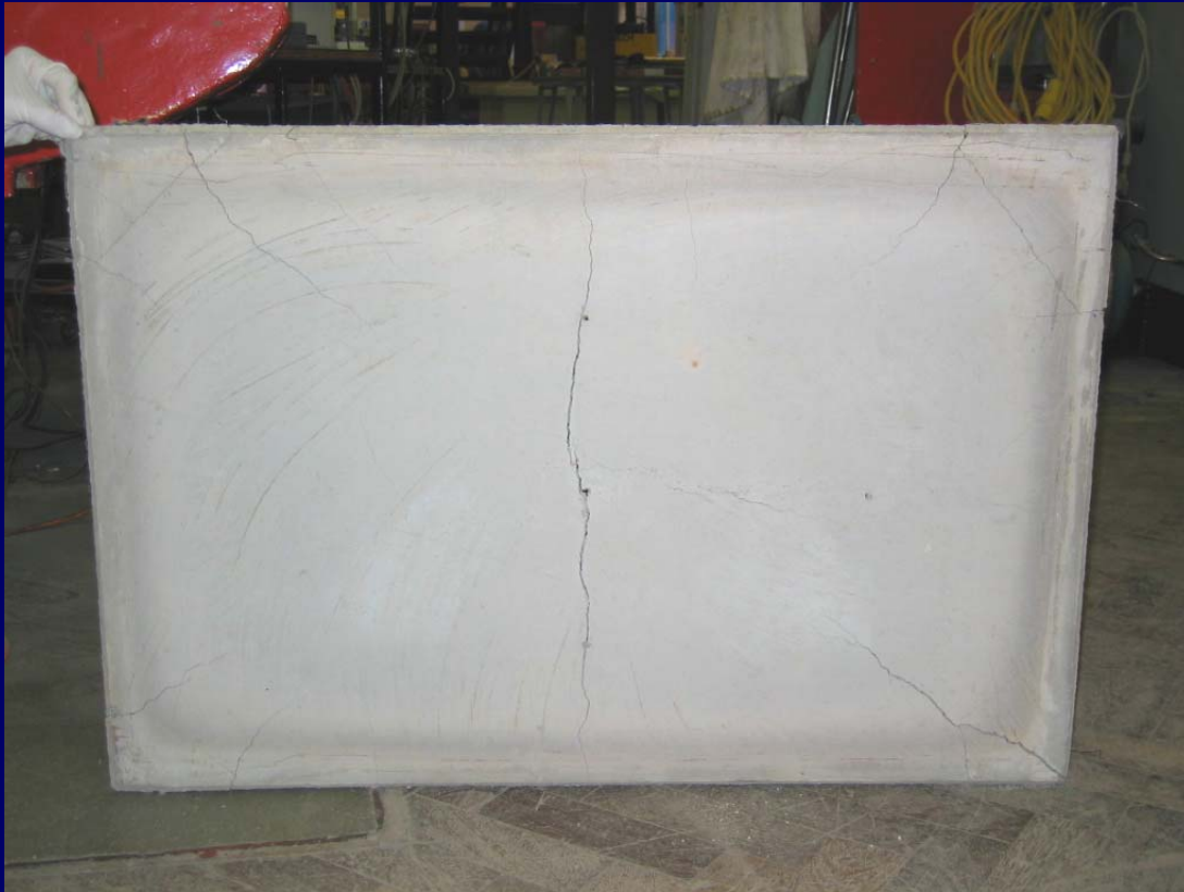
View of the underside of slab
