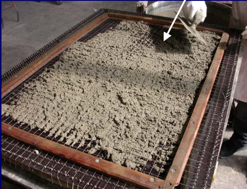
Casting the slab
